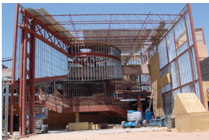
Construction of the Explora Science Museum staircase. Photo courtesy of Explora.
